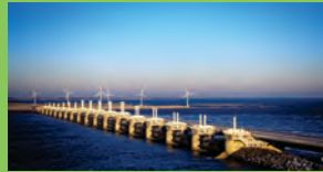
Eastern Scheldt Barrier , built with blast furnace slag cement with a design service life of 200 years
