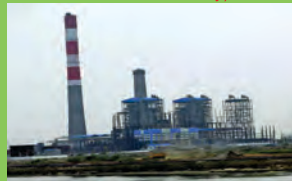
Thermal power project , Chennai
